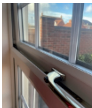
Window is open to allow ventilation but is still locked and secure.
